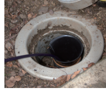
Insert Sleeve in cleanout
